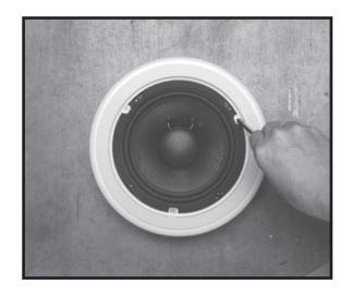
• Tighten the three screws at the front of your loudspeaker.
